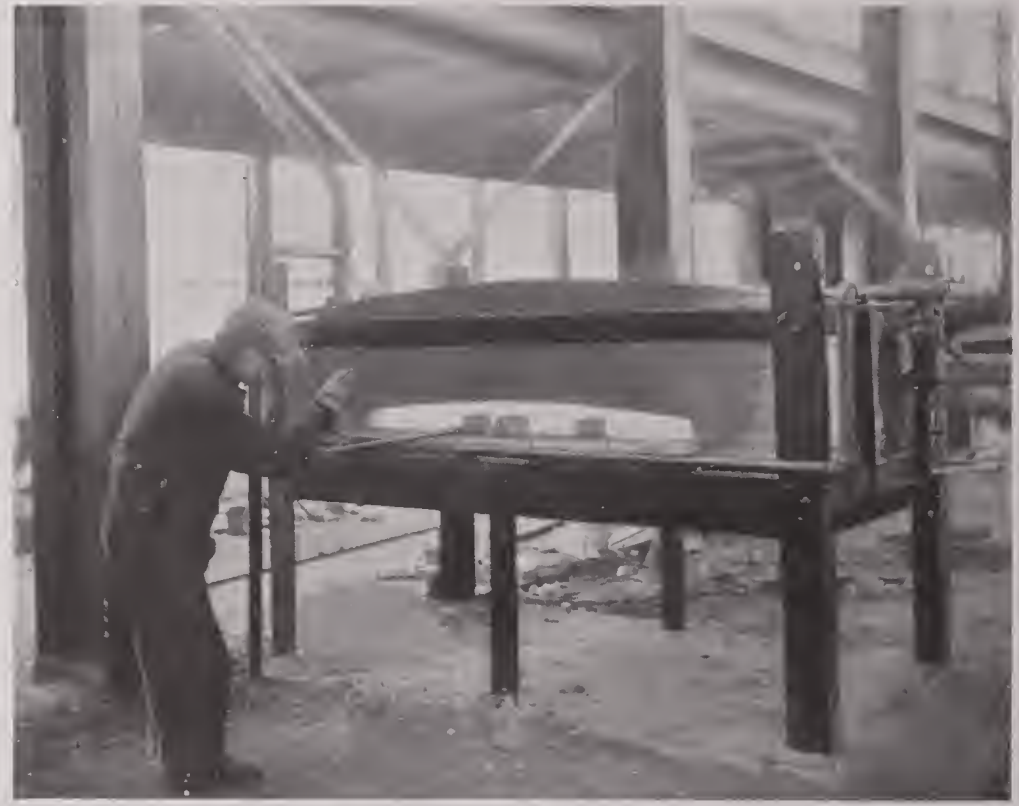
ONE OF THE FORGE SHOP FURNACES
